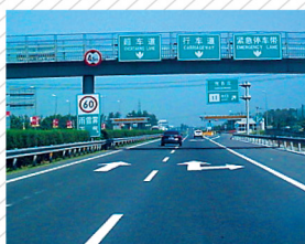
Ring Road to Beijing Int. Airport.
